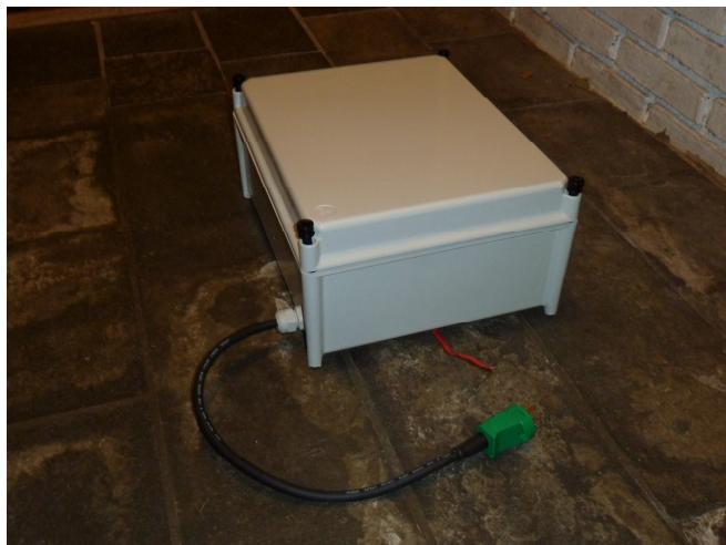
The box containing module for measuring temperatures, power supply and GSM-router.
